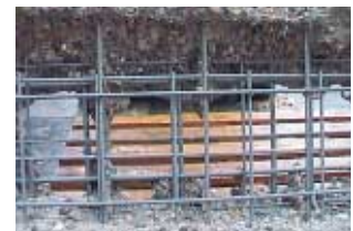
Concrete resurfacing and demolition with the URACA Vario Jet. The impressive demolition depth in hard concrete and the careful and efficient exposure of the reinforcement speaks for itself.
